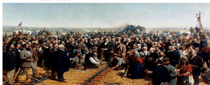
First Transcontinental Railroad completed in 1869: « Last Spike »
